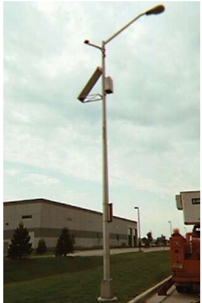
The collectors use solar panels to keep the batteries that operate the units charged.
